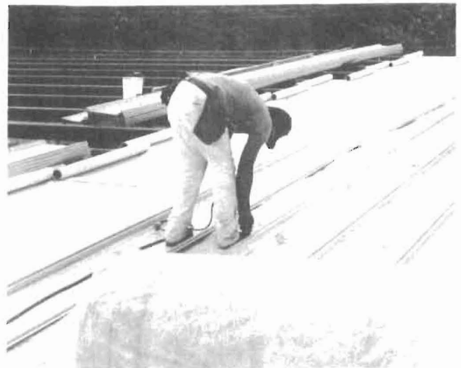
Figure 8. Foil-Elastomeric-Scrim-Kraft Vapor Retarder/Radiant Barrier; Emittance of 0.03.
