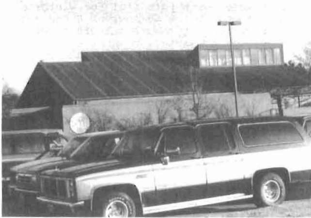
Figure 1. Exterior condensation on school roof assembly.
