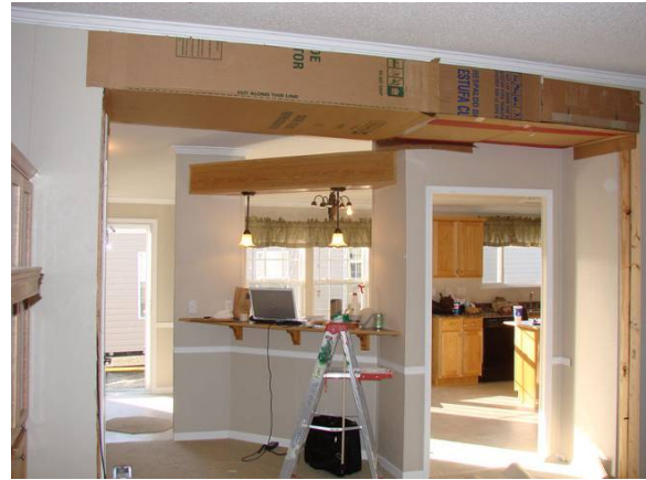
Figure 5 Southern Energy soffit mockup
