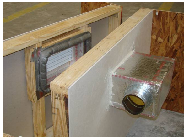
Figure 3 Southern Energy crossover mockup
