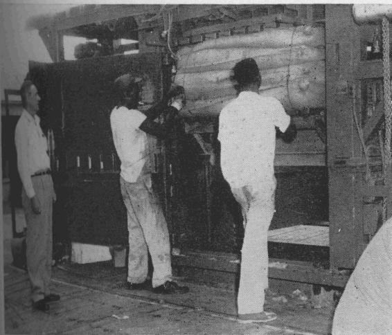
For shipment, original bags are compressed and wired. Courtesy: The Radio Post, Fredericksburg.
