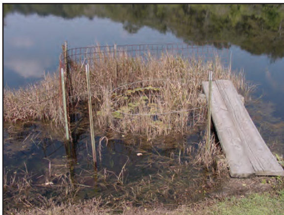
Figure 10. Use of fencing/cattle panels is the most effective means of excluding beaver from water control devices. Vegetation surrounding “pens” should be cleared periodically.
