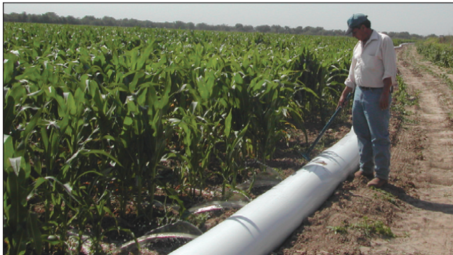
Figure 7. Using poly-pipe hole puncher.
