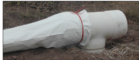
Figure 4b. Using rubber straps to connect the poly-pipe to the supplying pipe.
