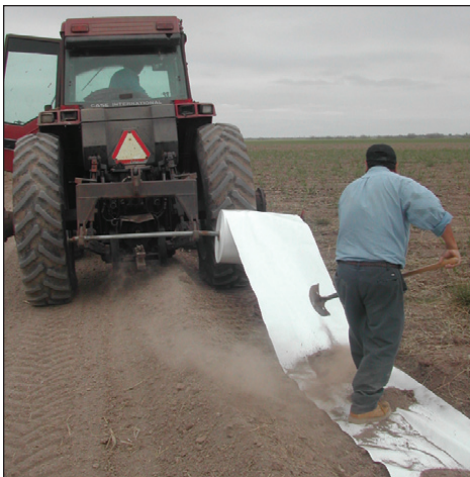
Figure 3. Placing dirt on poly-pipe at 10-foot intervals.
