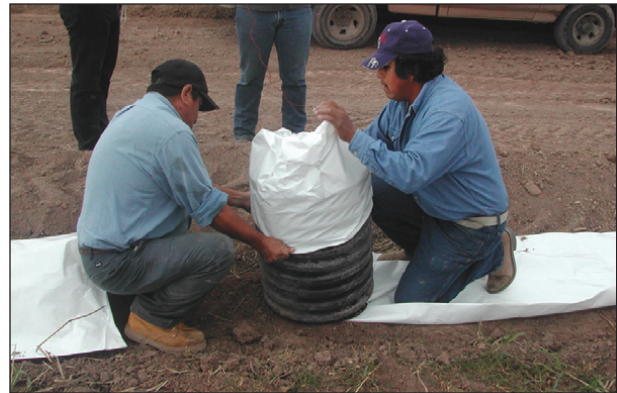
Figure 5a. Connecting two rolls of poly-pipe.
