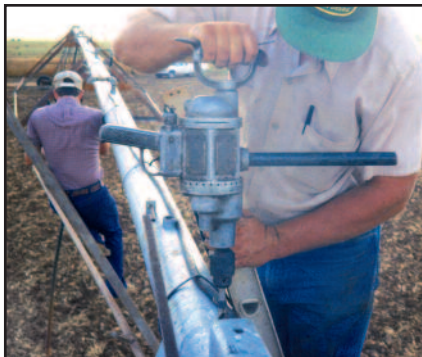
Figure 12. Drilling for swedge coupler.
