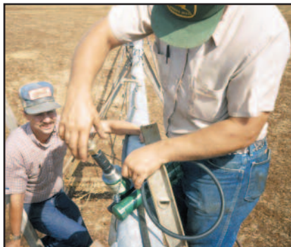
Figure 13. Installing swedge coupler.
