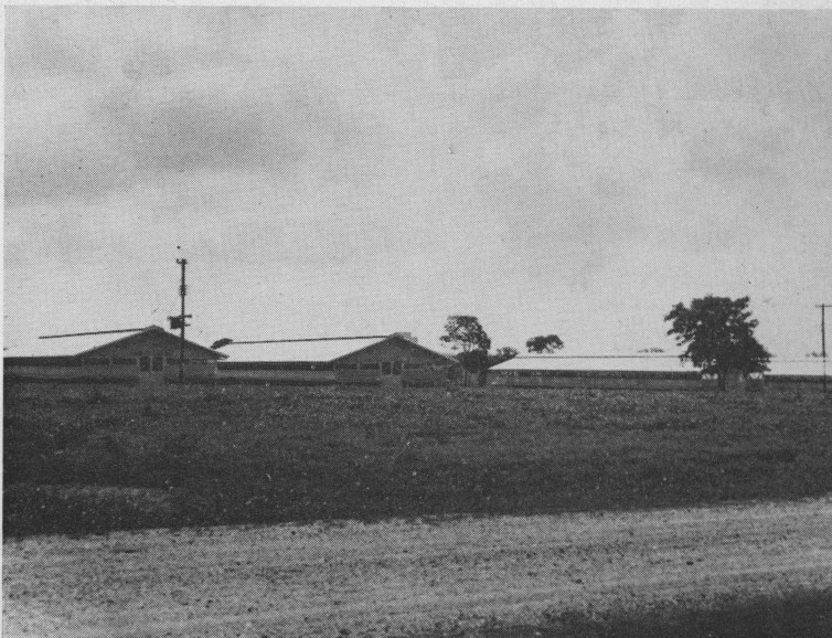
Figure 3. Houses with a continuous ridge row ventilator with roof line and floor line ventilator panels on the side walls.
