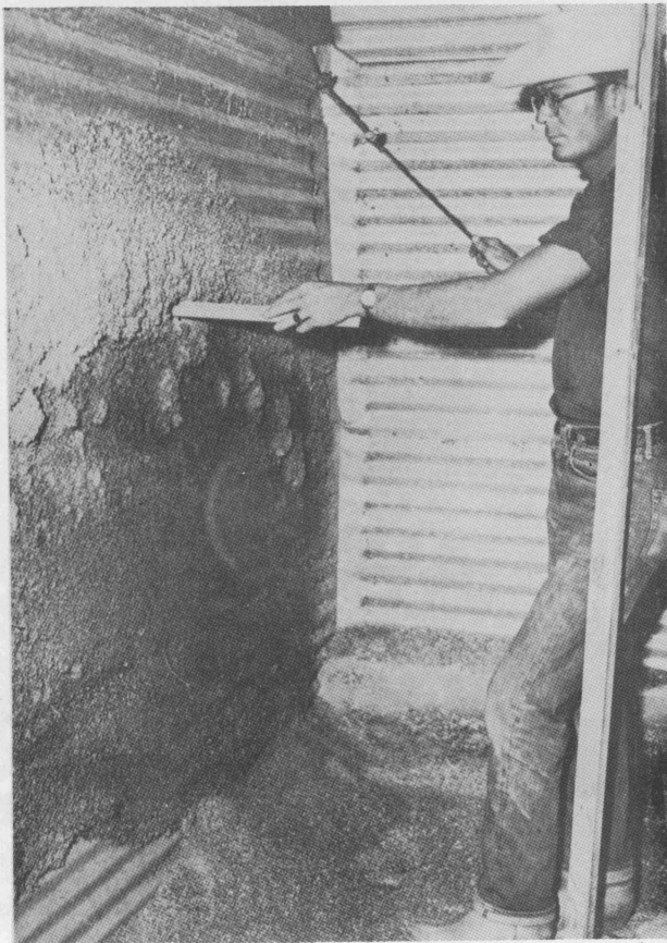
Figure 1. A tight structure is essential to prevent the entry of outside moisture. Moisture can cause high insect infestation and heating which result in considerable spoilage of grain.
