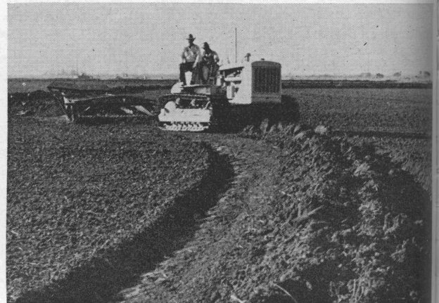
Figure 5. Building levees in a rice field.
