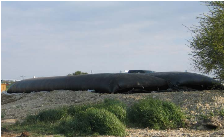
Fig. 2.b. Geotubes ® Filled to Approximately 5' in Height
