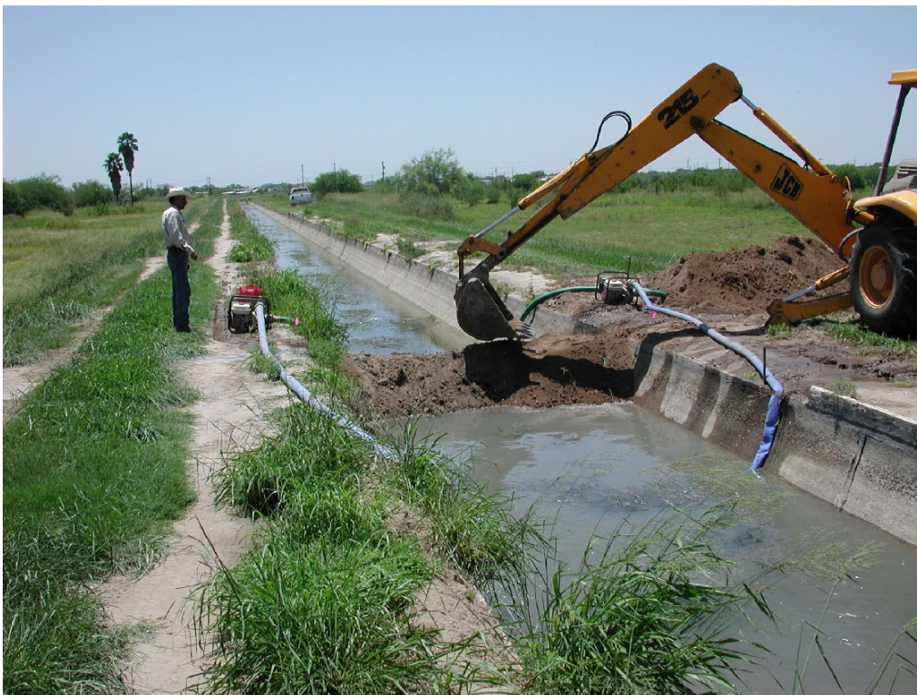
Figure 3. Photo of the earthen dam being built on test segment UN1.
