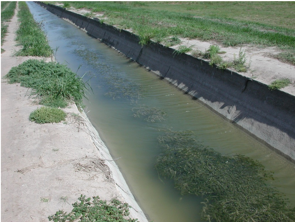
Figure 5. Photo of test segment UN1 showing aquatic vegetation problems.
