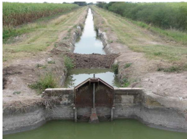
Figure 4. Lateral gate & earthen dam downstream
