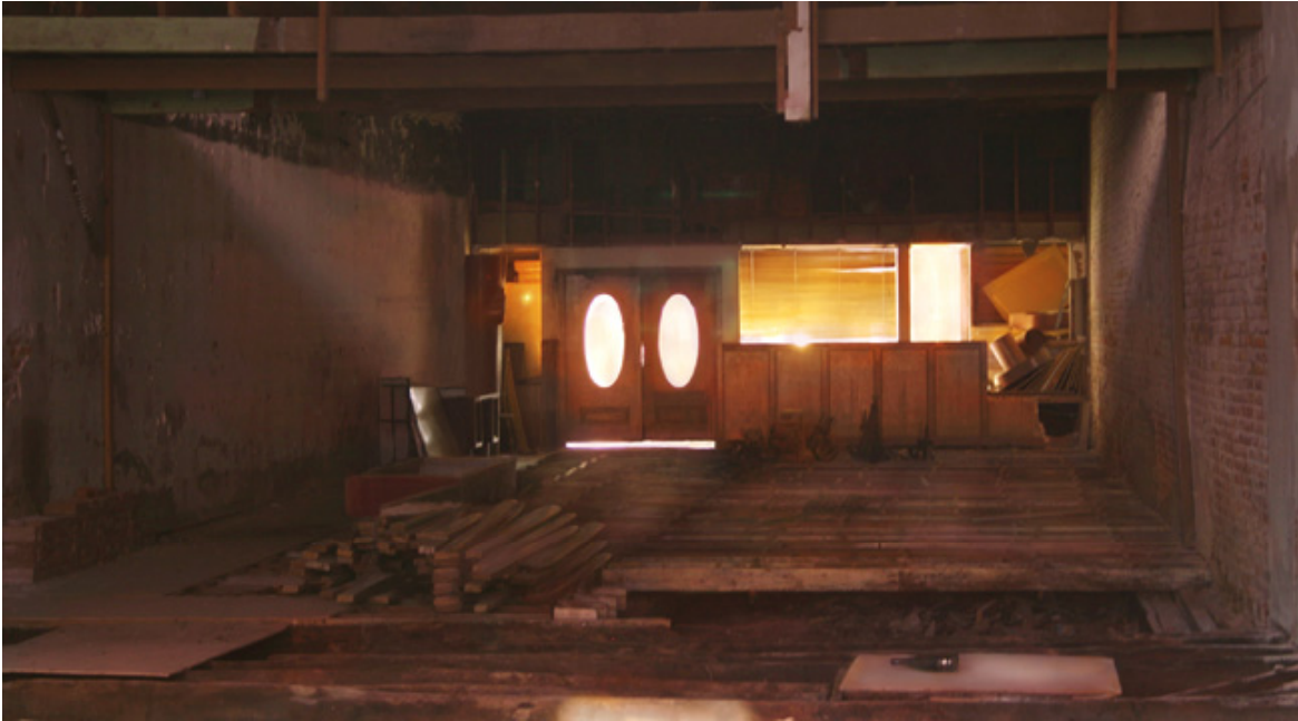
Figure 39. Case Study 5. Final Paint.
