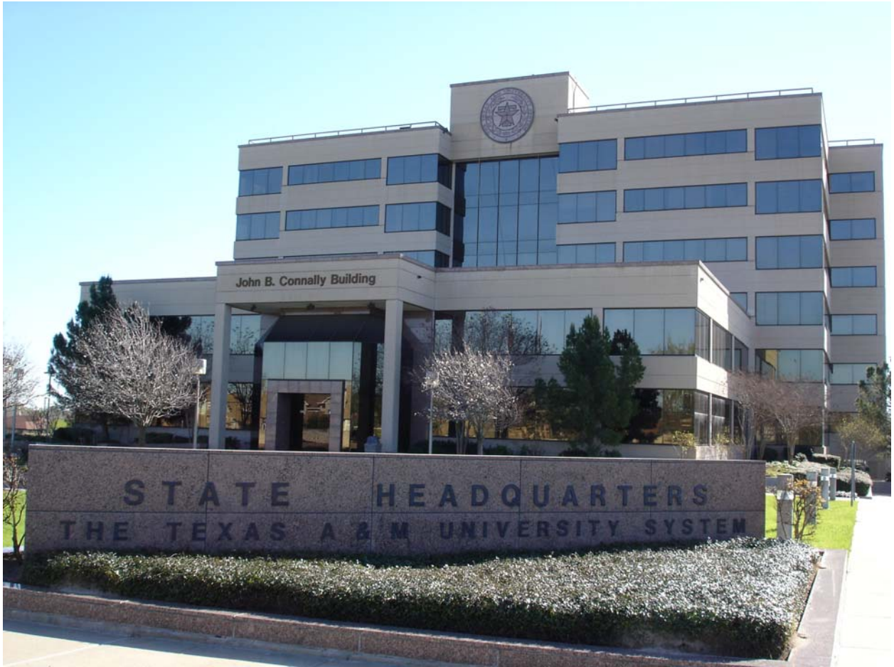
Figure 164: Standard Office Building (Texas A&M University Systems Building, College Station, Texas).
