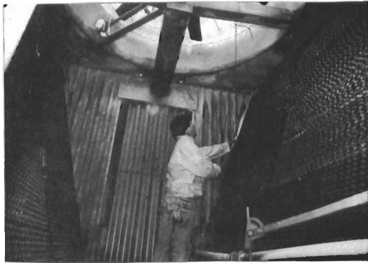
Figure 3 - Left, old-fashioned herringbone heavy wood slat drift eliminators with high static pressure loss which are prone to deterioration, permitting solid droplets of water to escape. Right, modern high efficiency low pressure drop, self-extinguishing PVC cellular eliminator replacements on typical crossflow tower.
