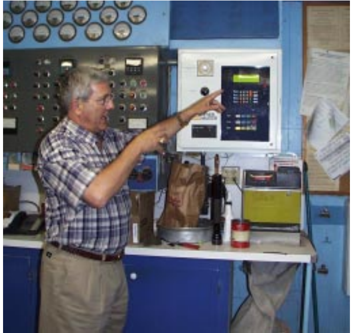
Dick explaining the new state-of-the-art computer system at the El Campo facility. The computer continually monitors grain moisture, and then makes heat and air flow adjustments as necessary to insure proper drying.
