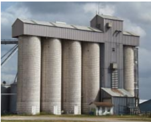
With the newly erected bins, the Gertson's have an on-farm storage capacity of 150,000 cwt of rice.
