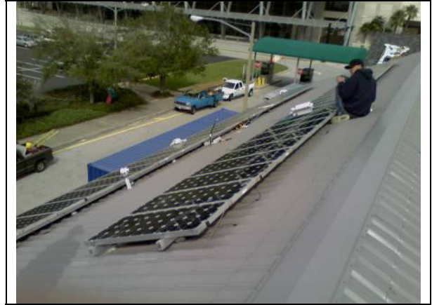
Figure 4 – 4.08 kW p PV system on Gen – X
