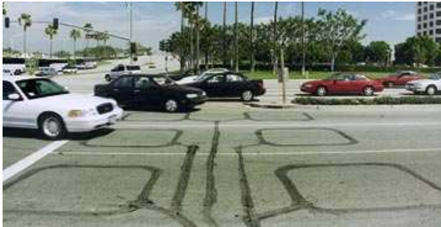
Fig. 3. Dual loop detector setup
