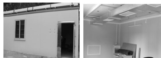
Fig.5 The photos of air-conditioning room for experimentation
