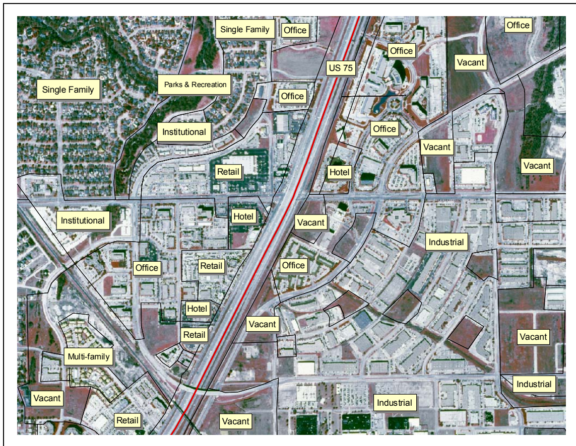
Figure 5.8 Aerial photograph of Telecom Corridor (part)
