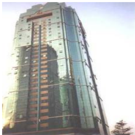
Fig.3 Huadu mansion building
