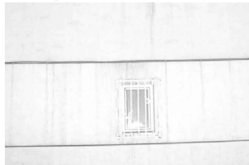
Fig.4 The correspondence photo with the thermographic image
