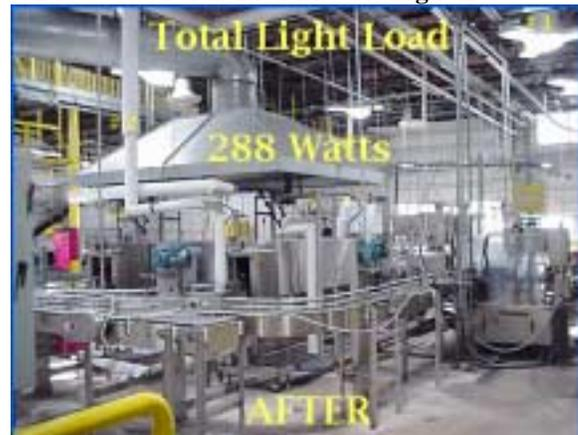
**AFTER**, Insulated Steam Lines, Steam Leaks Repaired and **Daylight Harvesting System** at a cost of **1. 99 Watts Per Lumen.**
