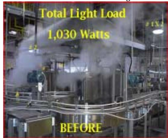
**BEFORE** 1 Non-Insulated Steam Lines, Steam Leaks and MH Lighting.
