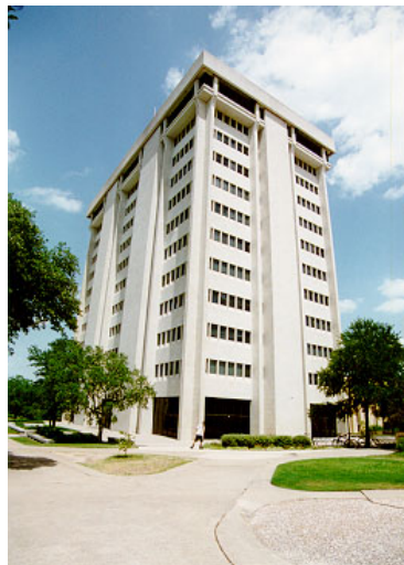
Figure 5.5 The Eller Oceanography and Meteorology Building on the Texas A&M University Campus.
