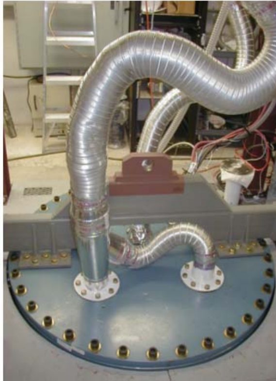
Fig. 50 Spin pit lid with test rig in pit
