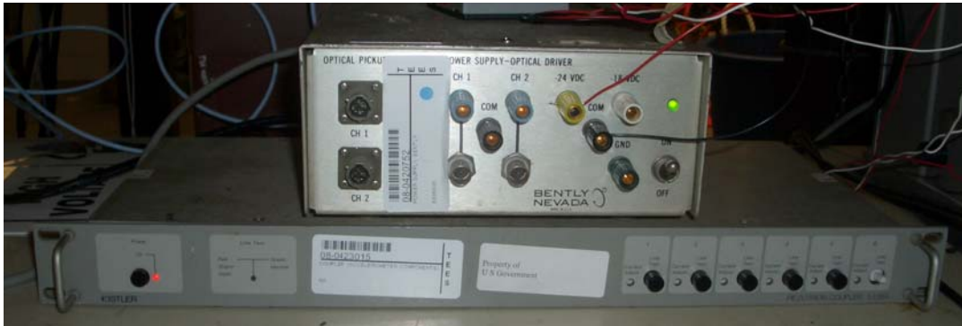
Fig. 45 Power supply for speed sensor (top) and accelerometers (bottom)
