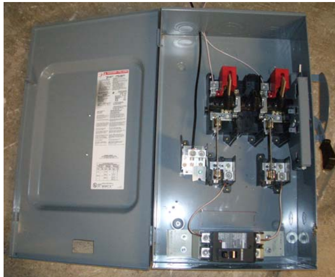
Fig. 57 Knife edge and breaker system
