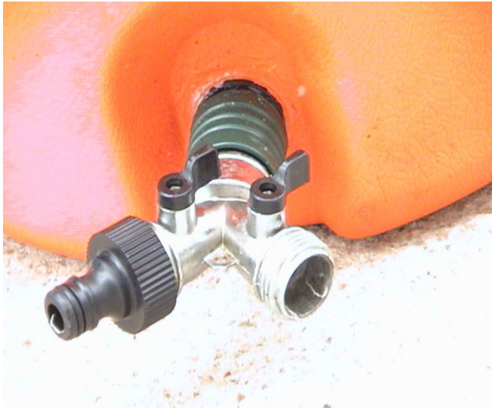
Figure 8 - Hose connector at the storage tank
