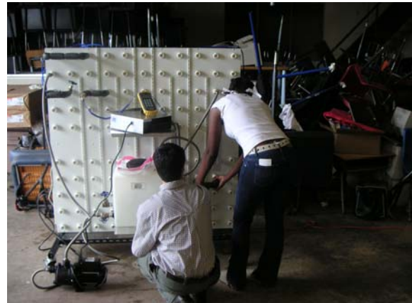
Figure 2. A middle school student attaching a control valve for a small-scale air conditioning system with the assistance of an undergraduate engineering student.
