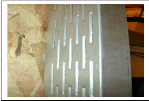
Figure 2. Steel stud with the slotted stud web.
