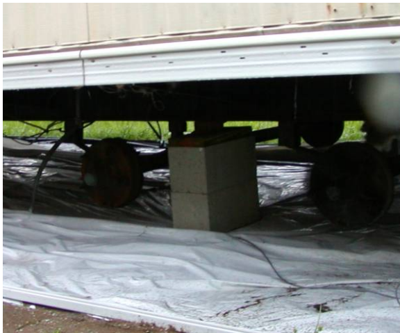
Figure 2 Ground Cover installed
