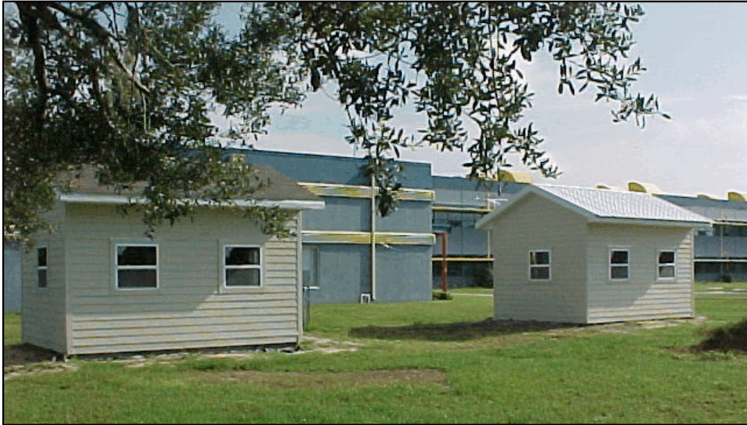
Figure 4. NightCool demonstration test buildings under construction
