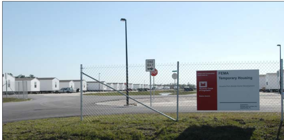
Figure 1. FEMA City, Arcadia, FL
