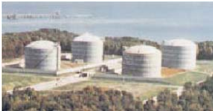
Fig. 6. Single Containment Tanks (UH IELE 2003b)
