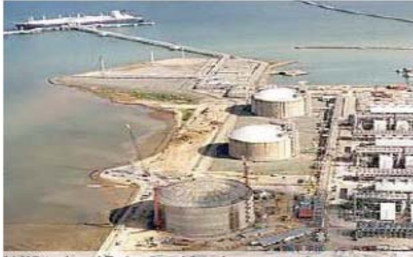
Fig. 7. Double Containment Tanks (UH IELE 2003b)
