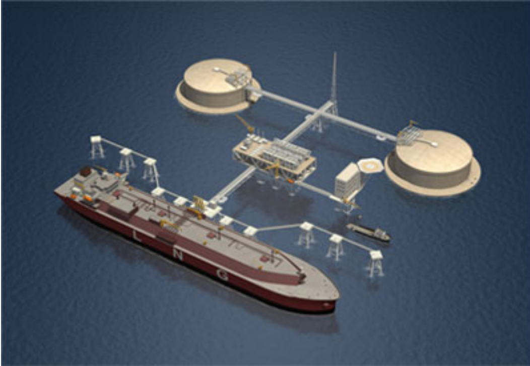
Fig. 25. LNG Terminal with Living Quarter That Is Located Outside of Hazardous Areas (Arup Energy 2004)
