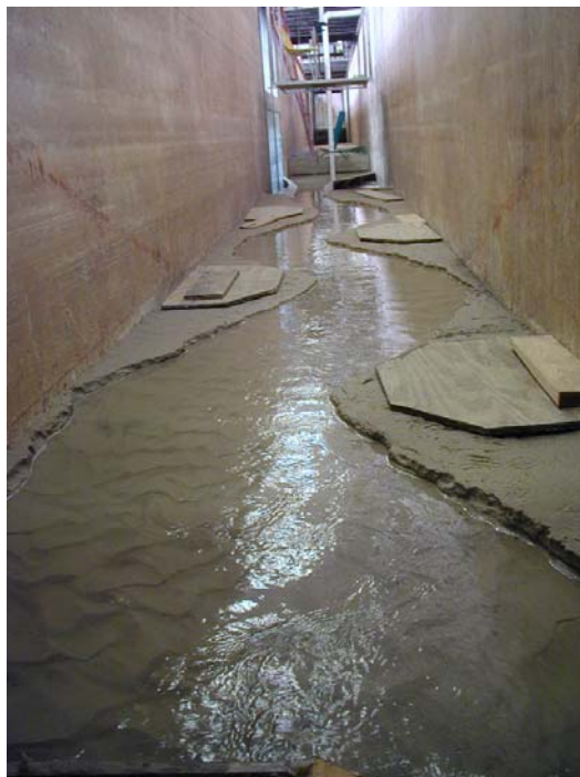
Figure B.18 Flume Test 10 at final stage, looking upstream
