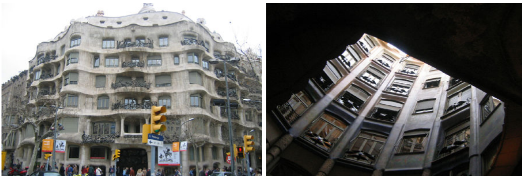
Figure 53. The façade and the enclosing walls around the patio (photographs by the author).
