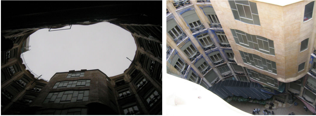
Figure 51. The interior patios of the Casa Mila (photographs by the author).
