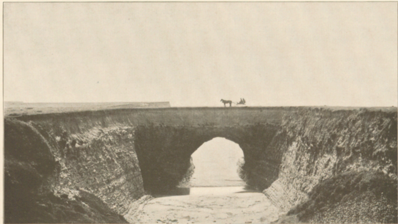
FIG. 6.—NATURAL BRIDGE IN MONTEREY SHALE, WHICH IS overlain BY 15 FEET OF QUATERNARY DEPOSITS FORMING THE SURFACE OF THE LOWEST MARINE TERRACE. On the coast, 3 miles west of Santa Cruz.
