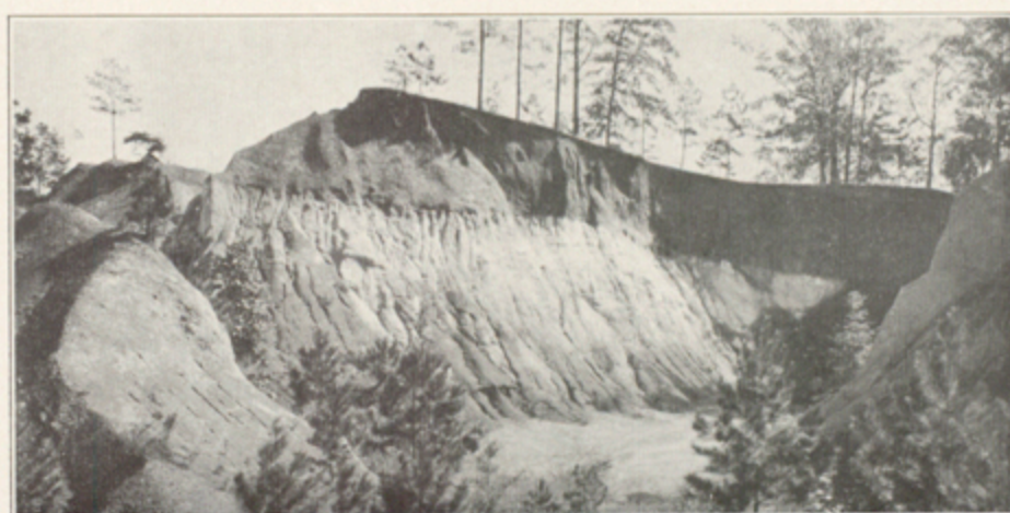
PLATE 11.—SHELBY IRON ORE DIGGINGS At top there is 15 feet of red loam carrying best quality of lump ore, underlain by light-colored sand and quartz gravel, possibly of Cretaceous age.
