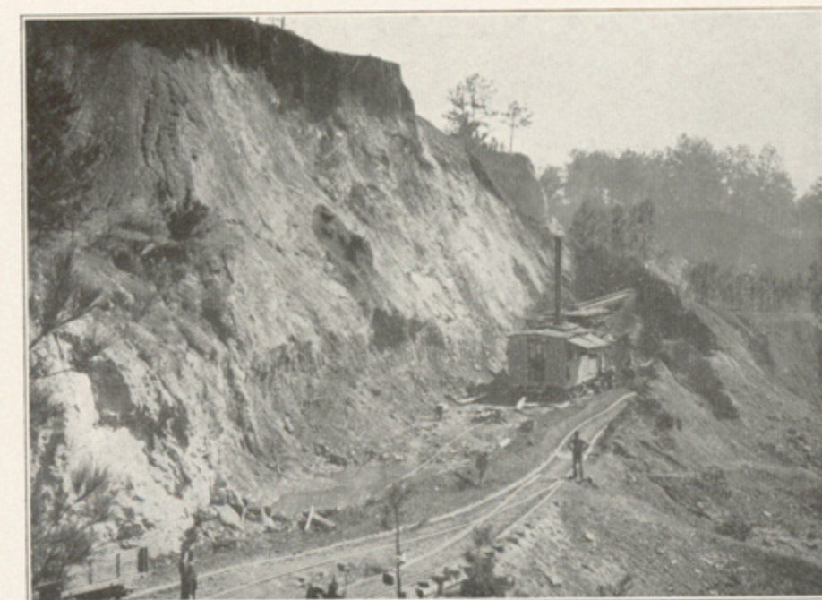
PLATE 15.—IRON ORE DIGGINGS AT SHELBY Ore is in pockets in decayed rock, which is reported to extend nearly 100 feet below the bottom of the pit. The clay seems to fill an ancient sink hole.
