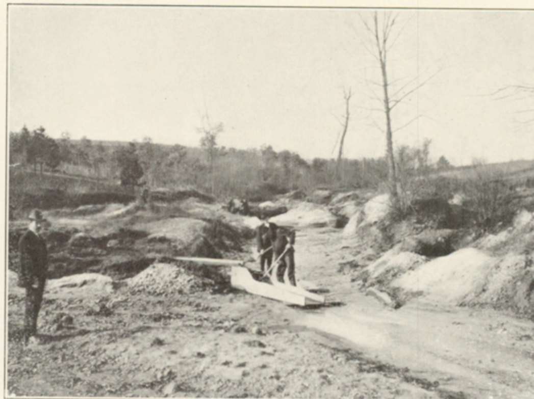
PLATE 8.—WASHING GRAVEL FOR MONAZITE, 4 MILES NORTHWEST OF GAFFNEY, S. C.
