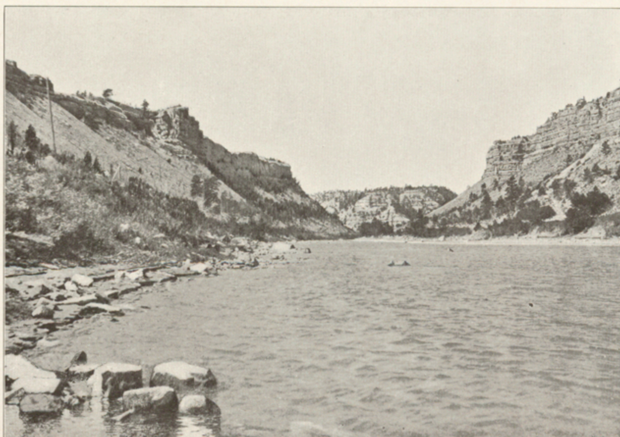
FIG. 5.—CANYON OF NORTH PLATTE RIVER, ONE AND ONE-HALF MILES ABOVE WENDOVER, LOOKING NORTHWESTERLY. A characteristic view of the canyon, which has been cut in the rocks of the Hartville formation.
