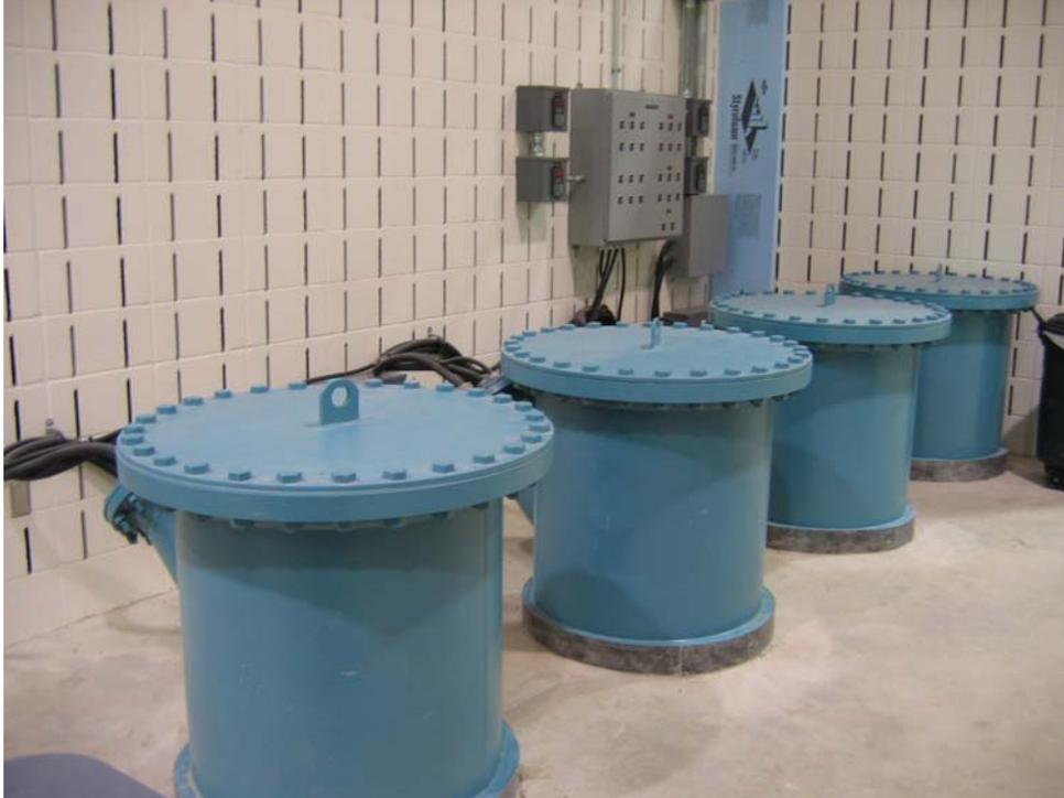
**Figure 6. Four pump heads**
