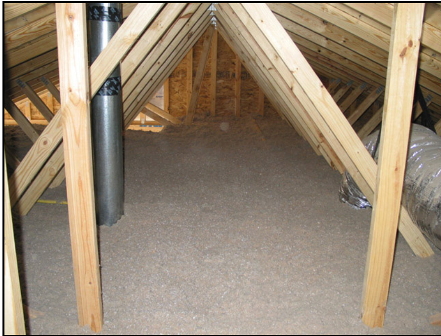
Figure 4.20 – Attic insulation
