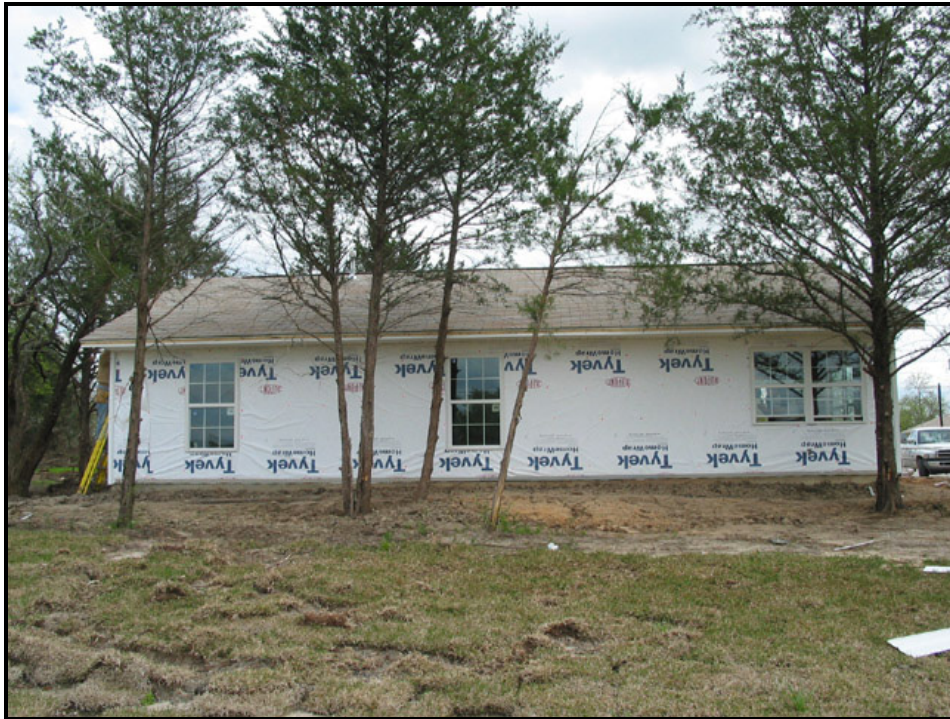
Figure 4.19 – Case study house (orientation – northwest)
