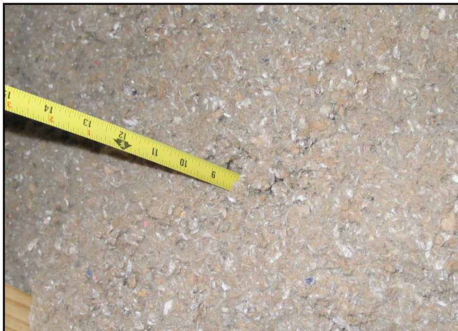
Figure 4.21 – Measuring the depth of the attic insulation
