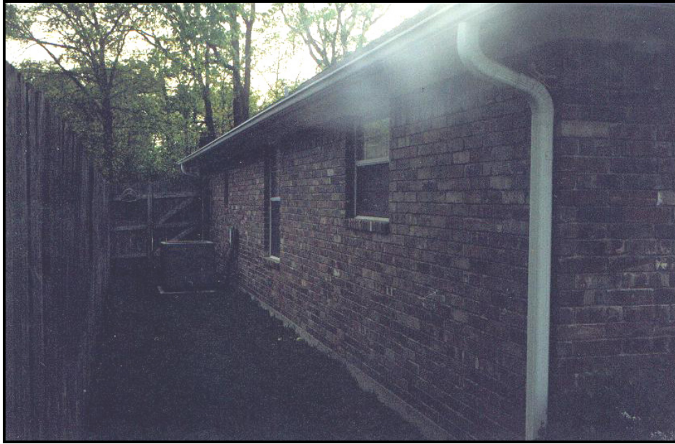
Figure 4.32 – Side of the case study house (northeast)
