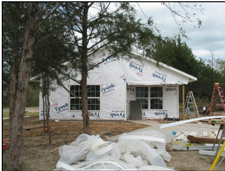
Figure 4.16 – Case study house (orientation – southwest)
