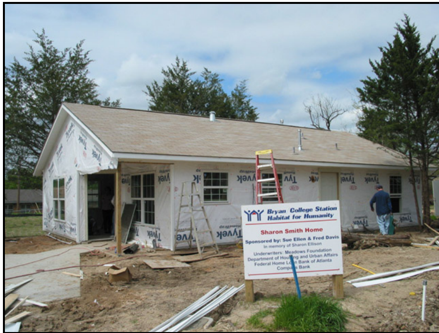
Figure 4.15 – Case study house: Habitat for Humanity, Bryan, Texas
