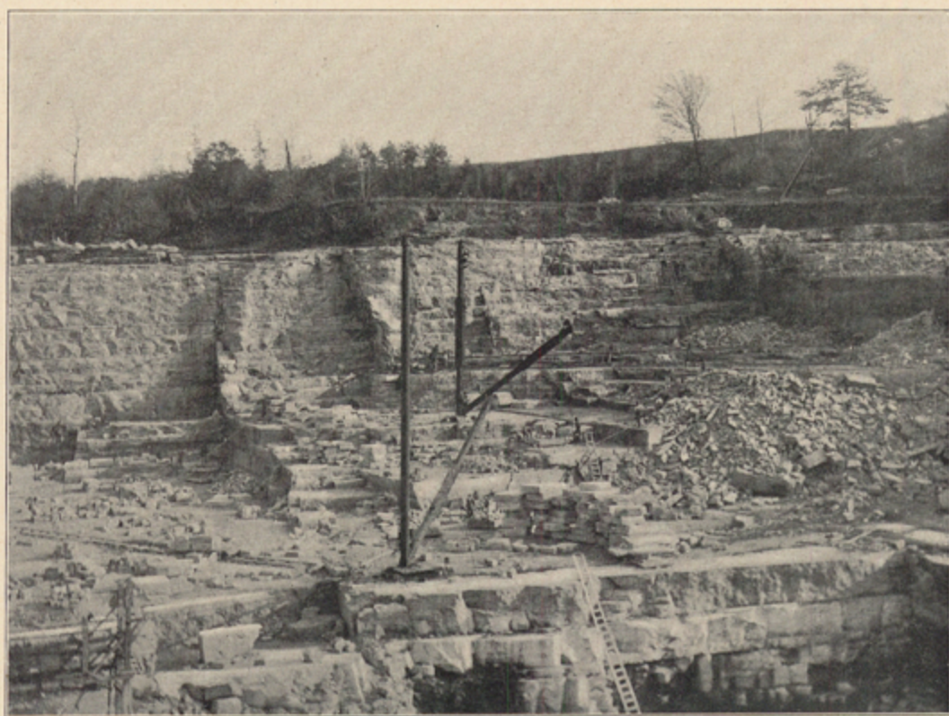
FIG. 12.—BUILDING-STONE QUARRY IN RACINE LIMESTONE AT WAUWATOSA, WIS.
