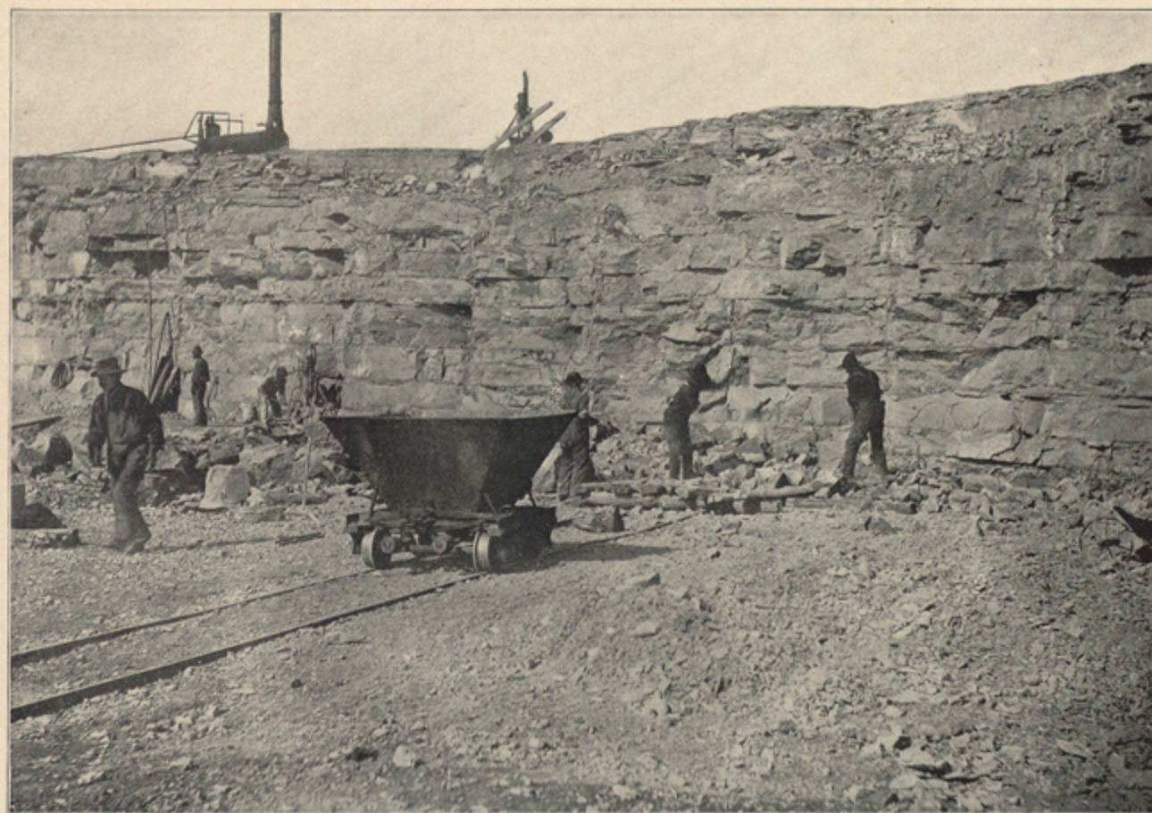
FIG. 13.—CEMENT-ROCK QUARRY IN MILWAUKEE FORMATION AT BERTHELET, JUST NORTH OF MILWAUKEE.
