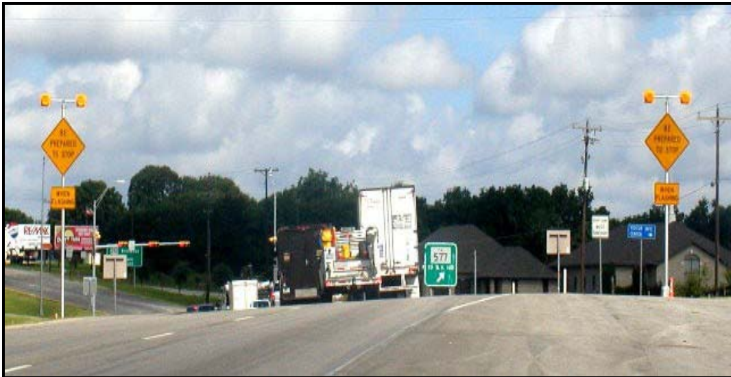
Figure 3.1 Westbound US 290 Approach in Brenham After AWEGS Installed
