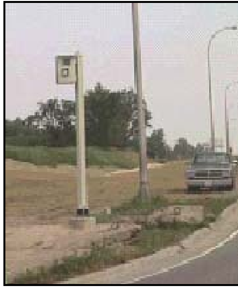
Figure 2.5 MIRS Pole and Camera Box
