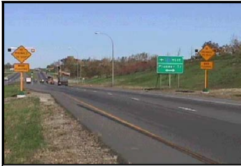
Figure 2.7 Advanced Warning Flashers on Trunk Highway 169 (34)
