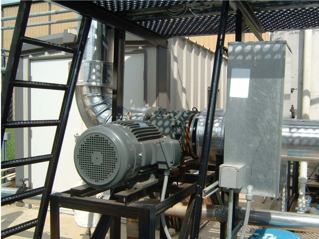
Figure A.32 The TVC method was supplemented with the Roots Blower to improve the performance. The Roots Blower was used to mechanically compress vapor before entering the jet ejector.
