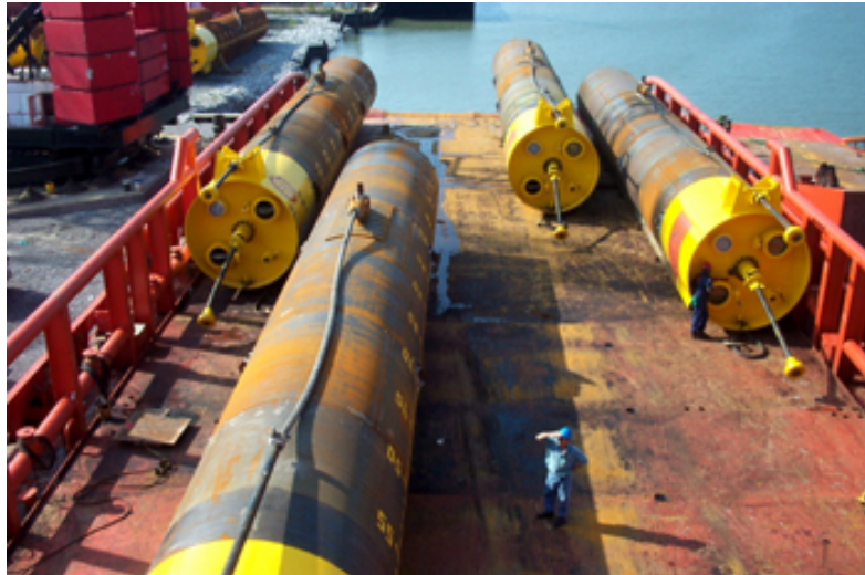
Figure 1.5 Suction caissons (Delmer)
