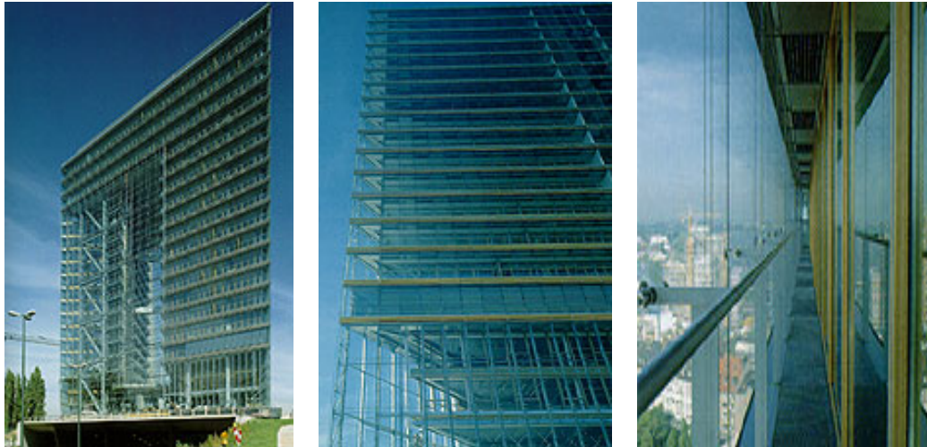
Fig. 13. Photographic Views of the Stadttor Building [17]
