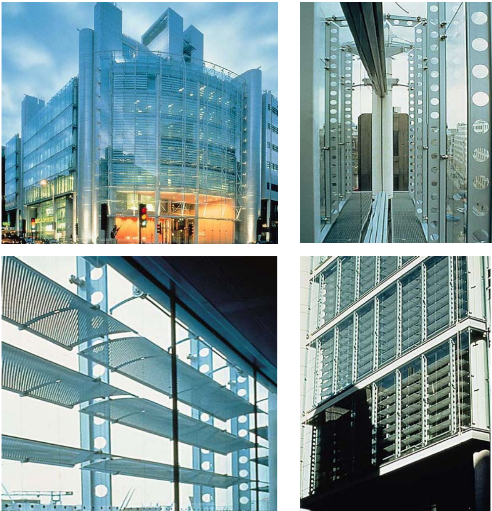
Fig. 10. Photographs of the Helicon Finsbury Building [24] Details of the facade and shading devices can be seen.
