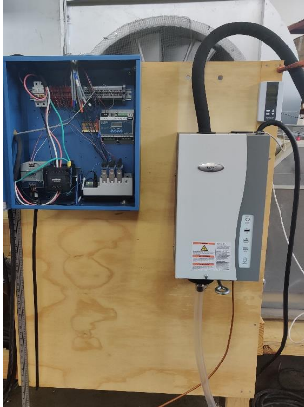
Figure 87: Humidifier Installation
