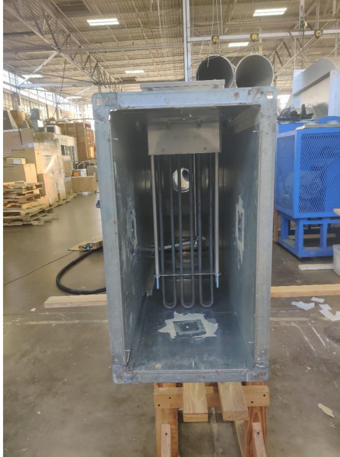
Figure 88: Process Heater Installation
