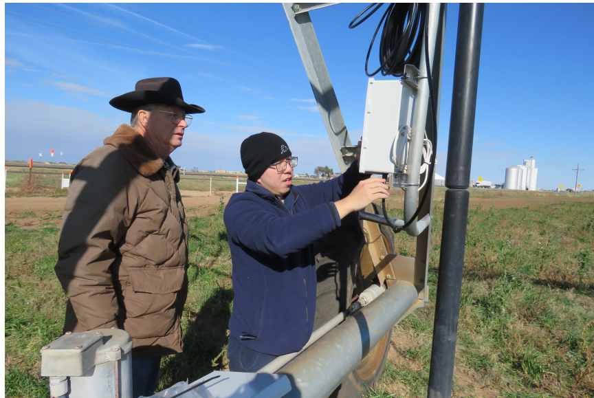
Figure 3.9: Communication system upgrade A, replacing previous Xbee module with more powerful one with external antenna.
