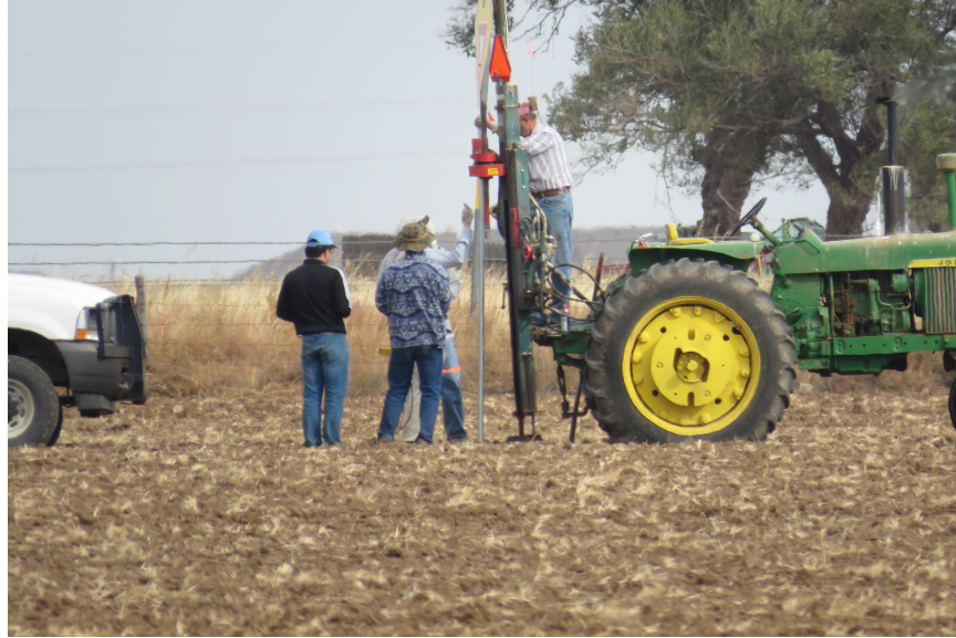
Figure 3.5: Digging holes in the field to deploy soil moisture sensors.
