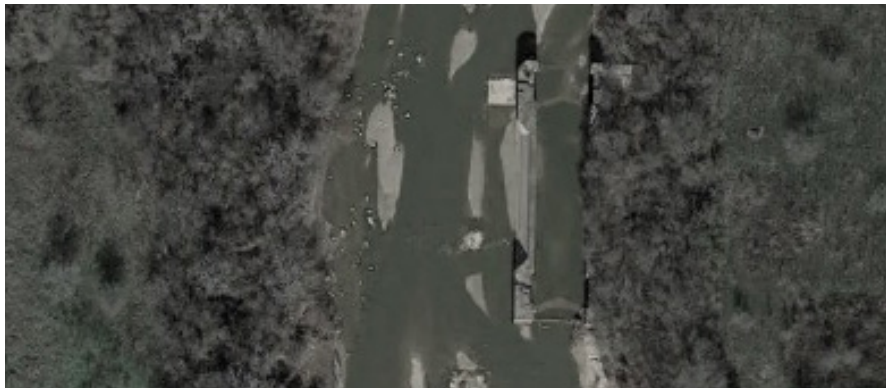
LOCK AND DAM #3
