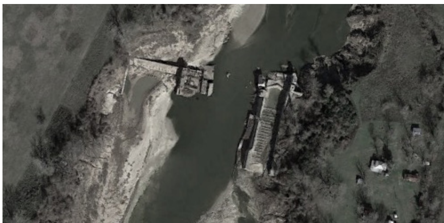
LOCK AND DAM #1
