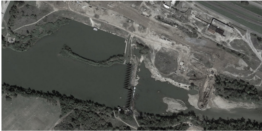
LOCK AND DAM #8
