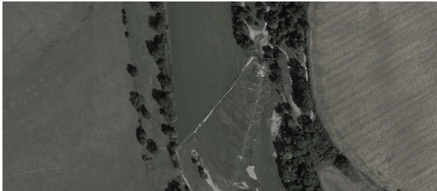
LOCK AND DAM #6
