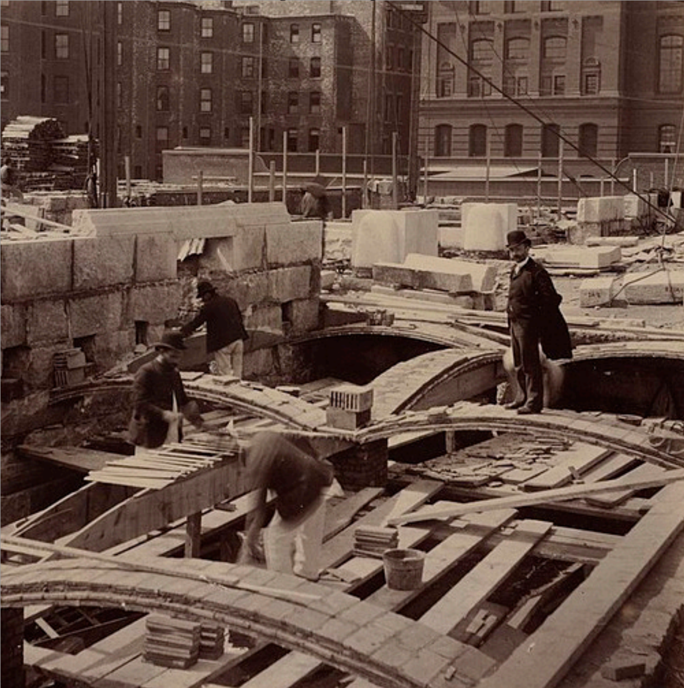
Rafael Guastavino, standing on a completed timbrel arch at a worksite.
