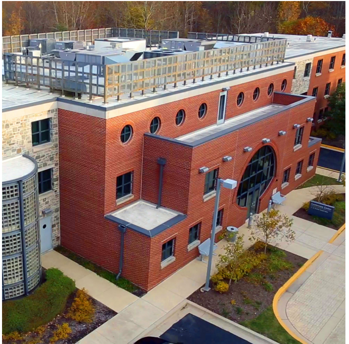
The International Masonry Training and Educational Facility in Bowie, MD.
